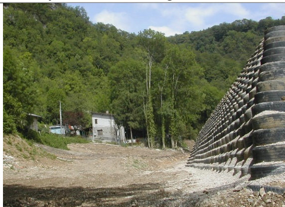
Merlon de protection – Saint Rambert
